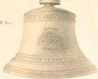
6 ft. DIAMETER. NOTE. C. Natural. Weight, 3 Tons, 7 Cwts, 3 Qrs, 24 Lbs.
