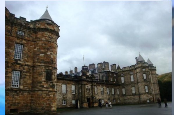
the Palace of Holyroodhouse.
