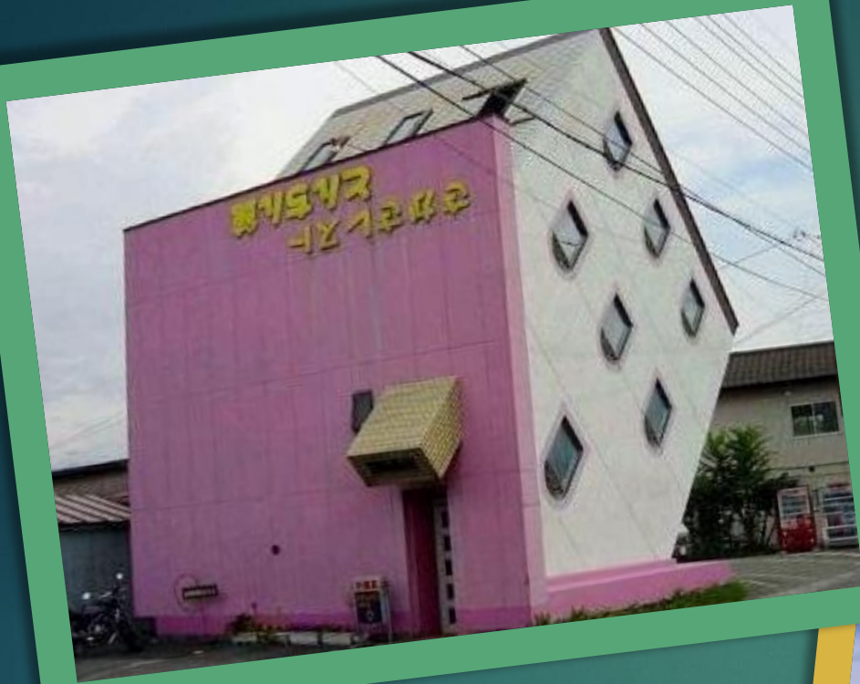
Tsunami House, Japan
