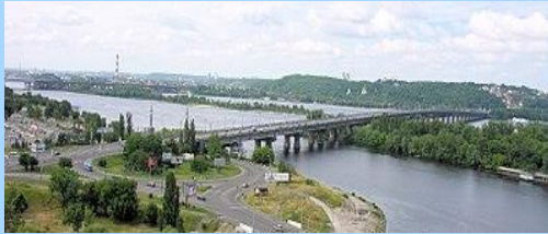
The Paton Bridge is the world's first all-welded bridge. Kiev. 2008
