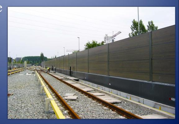
However, if the rail noise can not be reduced in origin, then the solution is in noise barriers. They should be placed as close as possible
