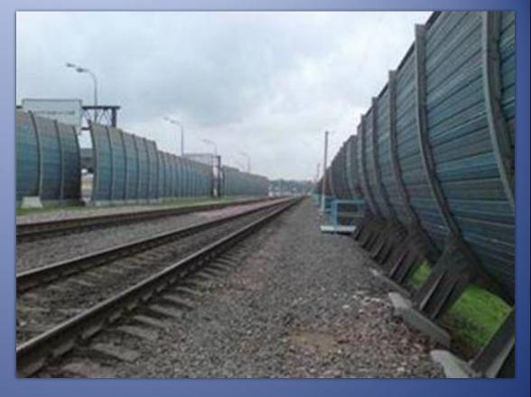
to the track and have a height no less than 2 meters. In addition noise barriers should be made of special absorbing materials for additional noise reduction.
