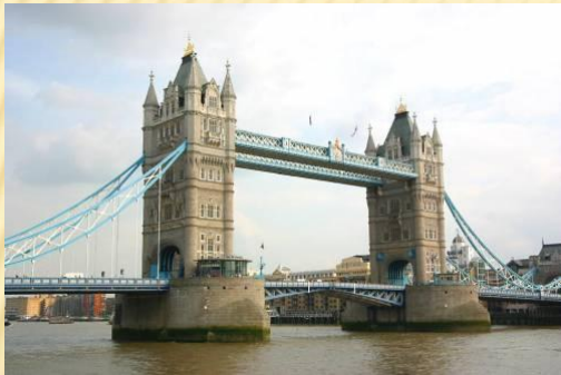
a) Tower Bridge
