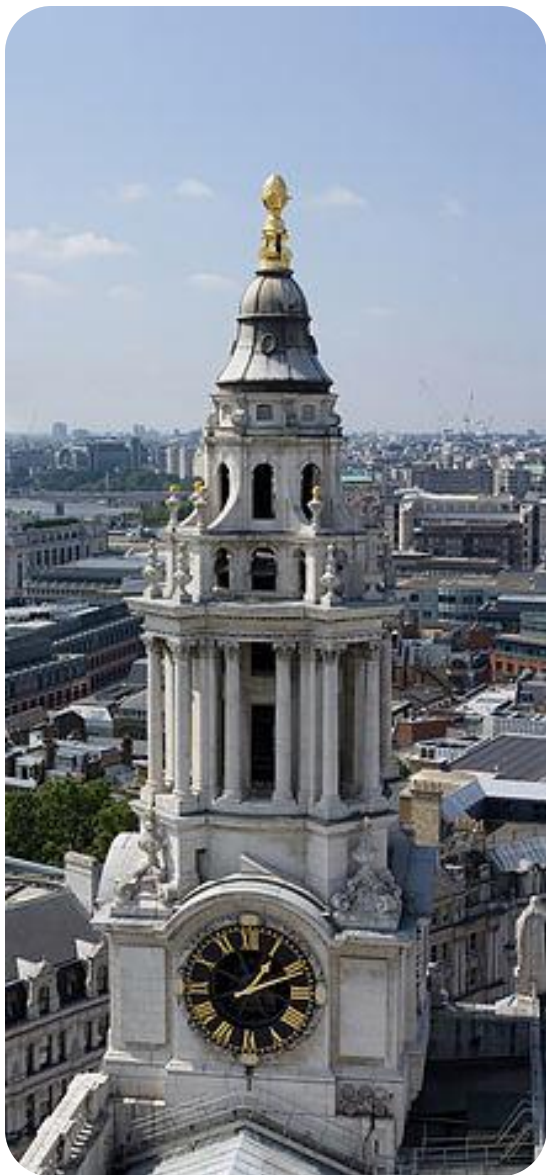
South west tower of St. Paul's Cathedral.
