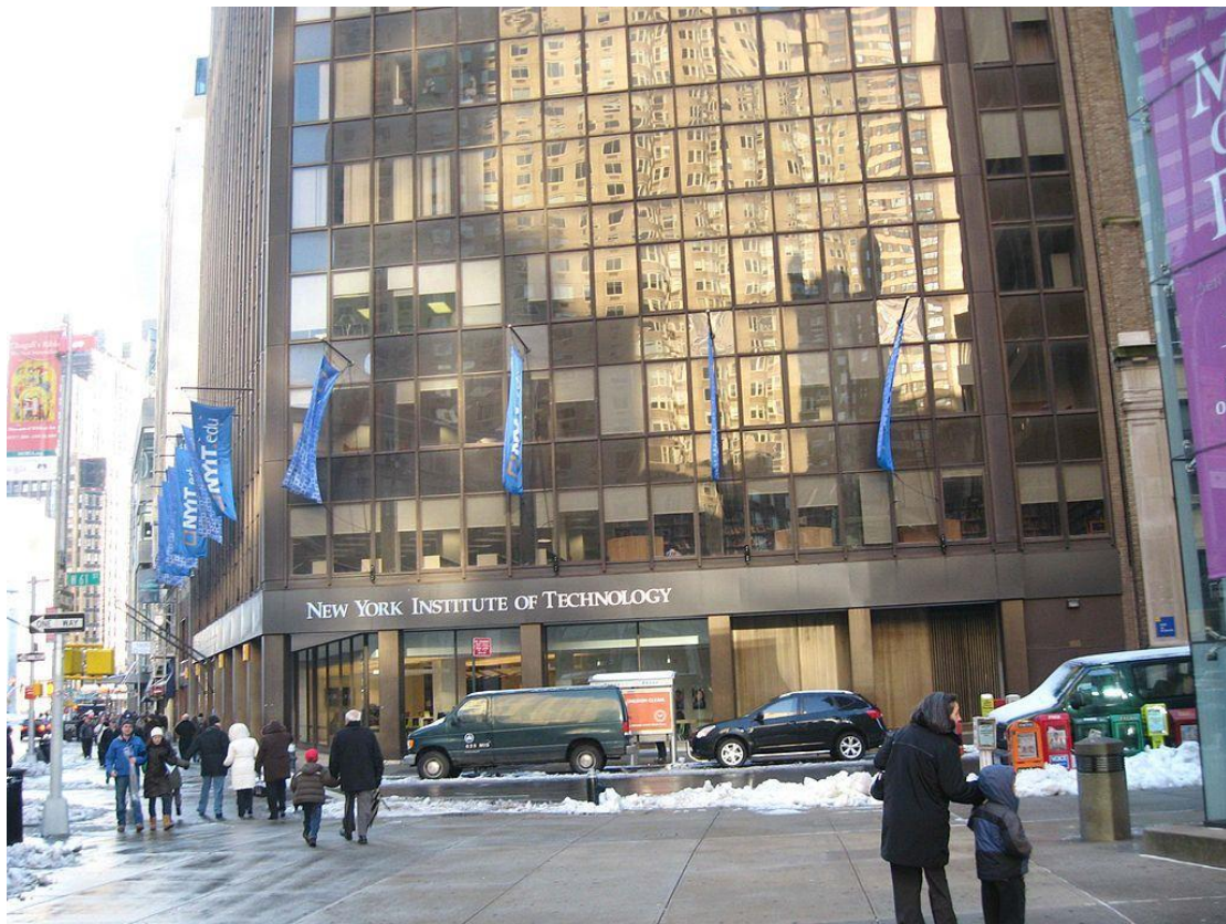
A building of New York Institute of Technology on its Manhattan campus
