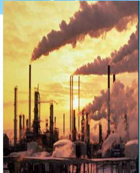
Burning of fossil fuels Power plant exhausts Producing carbon dioxide
