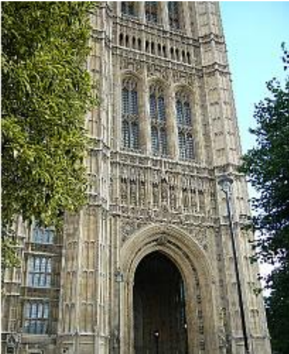
The Sovereign's Entrance at the bottom of Victoria Tower
