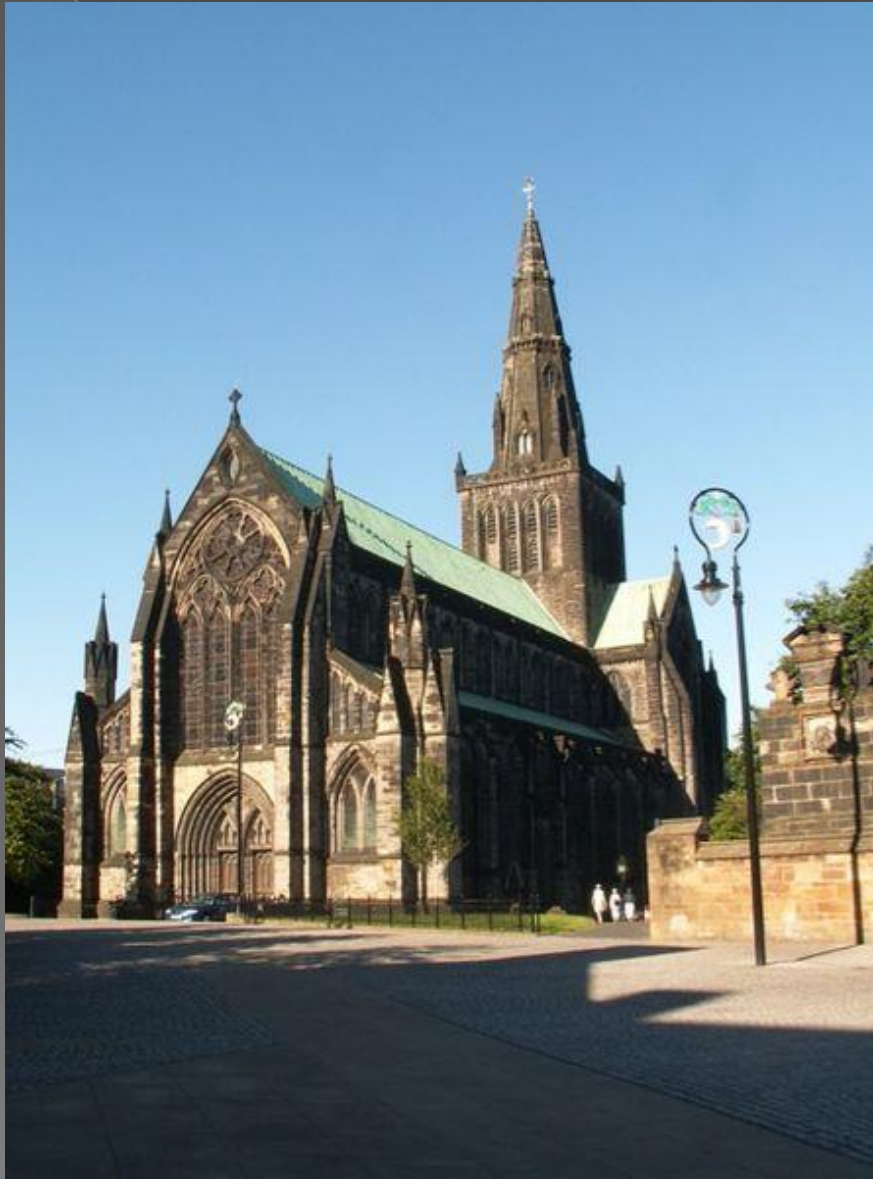
St. Mungos Cathedral
