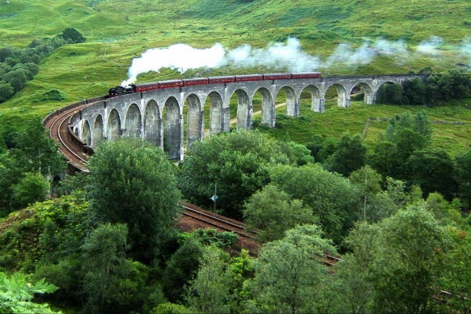
Glennfinnan Viaduct, Scotland
