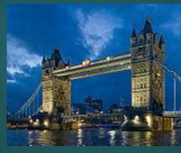
The bridge consists of two towers which are tied together at the upper level by means of two horizontal walkways which are designed to withstand the horizontal forces exerted by the suspended sections of the bridge on the landward sides of the towers. The bascule pivots and operating machinery are housed in the base of each tower. The bridge's present colour dates from 1977 when it was painted red, white and blue for the Queen's Silver Jubilee. Originally it was painted a chocolate brown colour.
