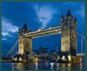
The bridge consists of two towers which are tied together at the upper level by means of two horizontal walkways which are designed to withstand the horizontal forces exerted by the suspended sections of the bridge on the landward sides of the towers. The bascule pivots and operating machinery are housed in the base of each tower. The bridge's present colour dates from 1977 when it was painted red, white and blue for the Queen's Silver Jubilee. Originally it was painted a chocolate brown colour.
