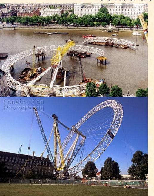
In the process over 1700 tons of steel were used for the structure and more than 3000 tons of concrete were used for the foundations. Its steel design forms an "A" shape, with two large tapered legs at the base -20 meters apart and each over 58 meters in length. The legs lean toward the river at a 65-degree angle. The rim of the Eye is supported by tensioned steel cables and resembles a huge spoked bicycle wheel.
