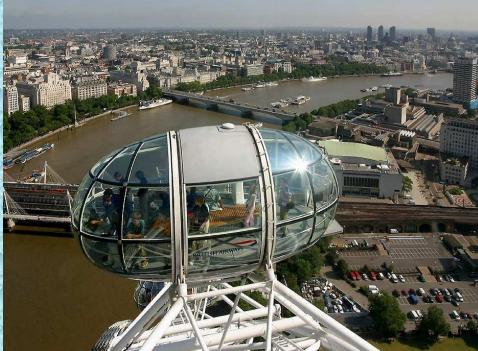
The wheel's 32 sealed and air-conditioned ovoidal passenger capsules are attached to the external circumference of the wheel and rotated by electric motors. Each of the 10-tonne capsules represents one of the London Boroughs, and holds up to 25 people, who are free to walk around inside the capsule, though seating is provided. The wheel rotates at 26 cm per second so that one revolution takes about 30 minutes.
