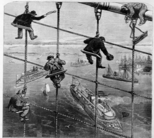
NEW YORK.—COMPLETING A GREAT WORK.—LASHING THE CHAINS OF THE BROOKLYN BRIDGE. Photo & Engraving by a Great Artist.—THE BUREAU.
