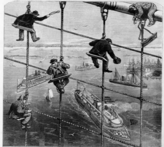
NEW YORK.—COMPLETING A GREAT WORK.—LASHING THE CHAINS OF THE BROOKLYN BRIDGE. FROM A SKETCH BY A GREAT ARTIST.—THE BUREAU.
