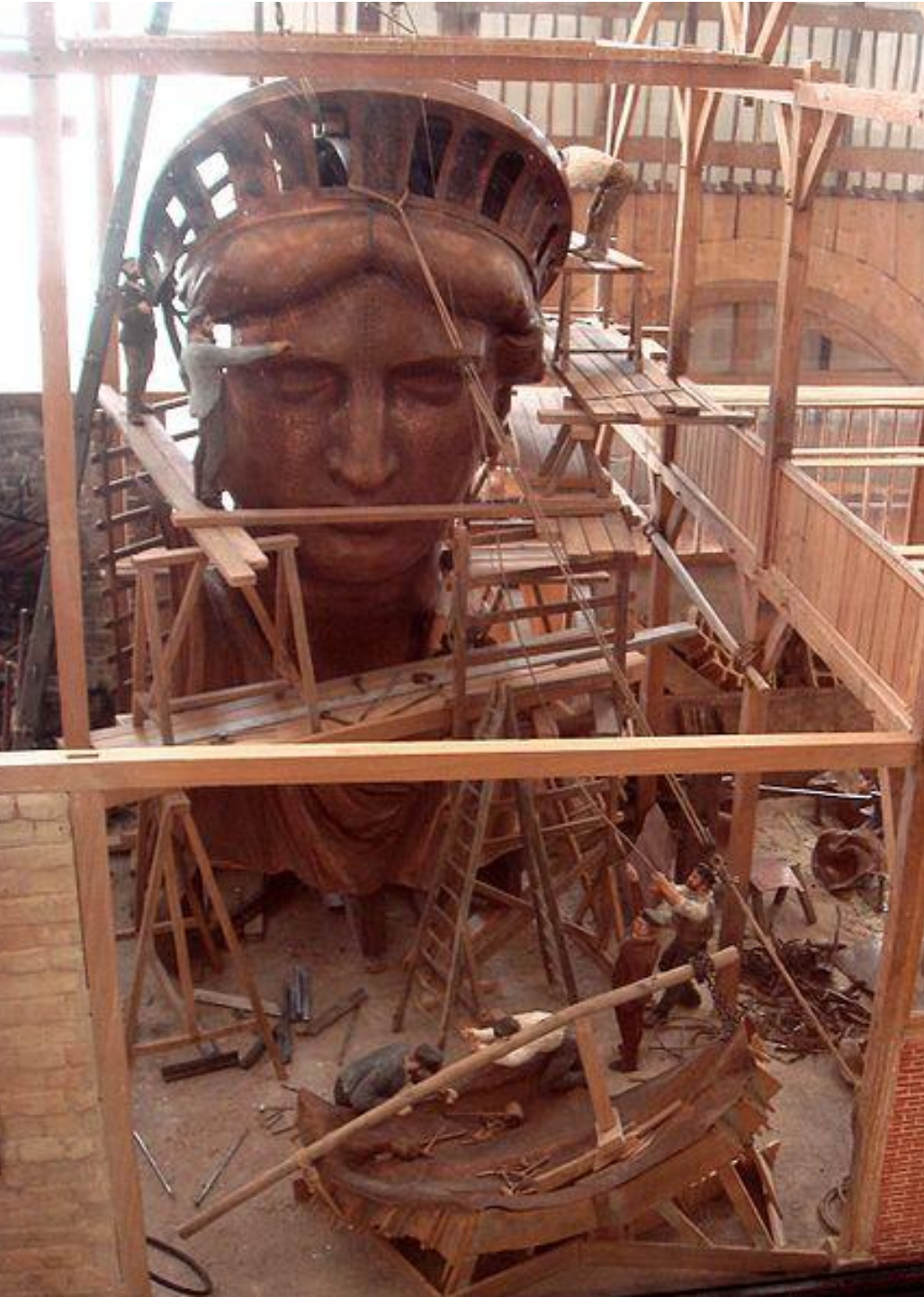
Diorama of the manufacture of Liberty's copper head in the ateliers of Gaget, Gauthier and Cie
