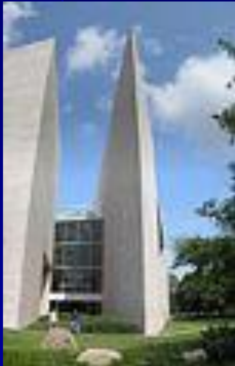
Detail of the corner of the East Building
