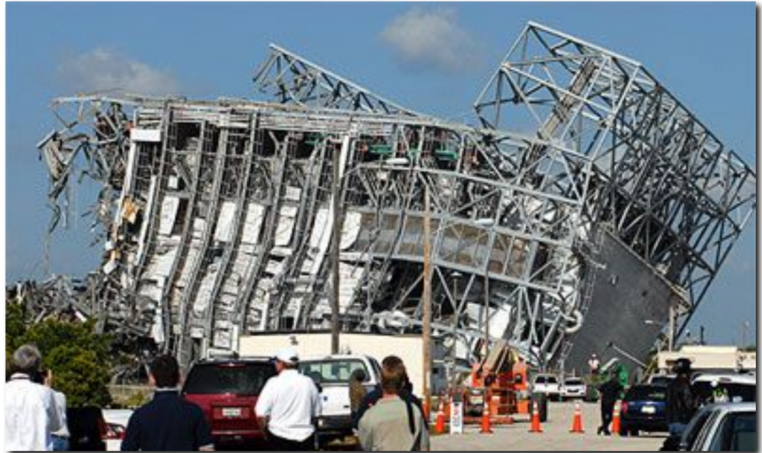
Demolition of legacy Mobile Service Tower (27 April 2008)
