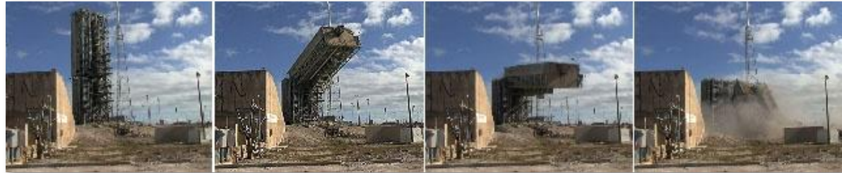
Demolition of legacy Umbilical Tower (8 January 2008)
