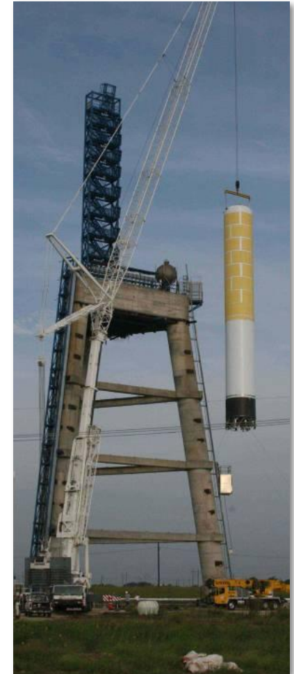
Raising first stage tank on to test stand
