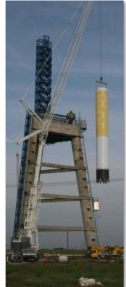
Raising first stage tank on to test stand
