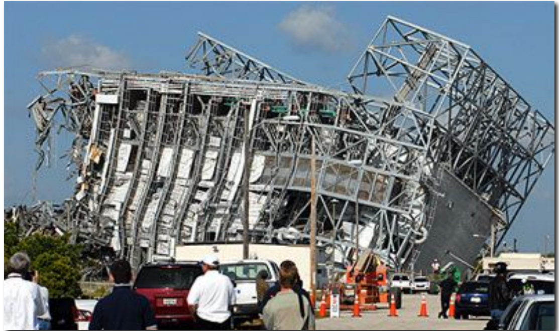
Demolition of legacy Mobile Service Tower (27 April 2008)
