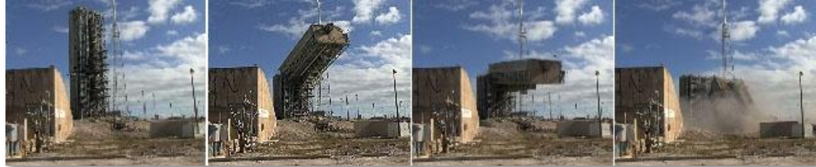
Demolition of legacy Umbilical Tower (8 January 2008)
