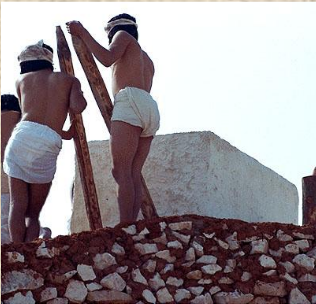
Rocking a block into position
