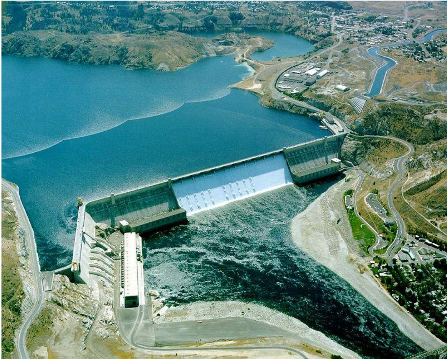
Grand Coulee Dam in Washington
