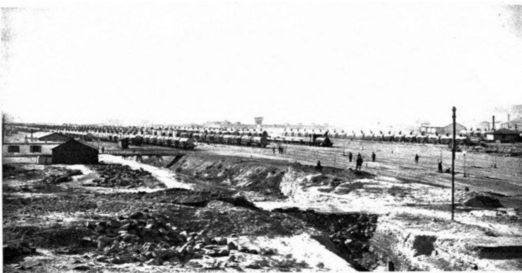
FIG. 84.—TANK CARS ON RAILWAY SIDINGS NEAR BLACK TOWN, BAKU.
