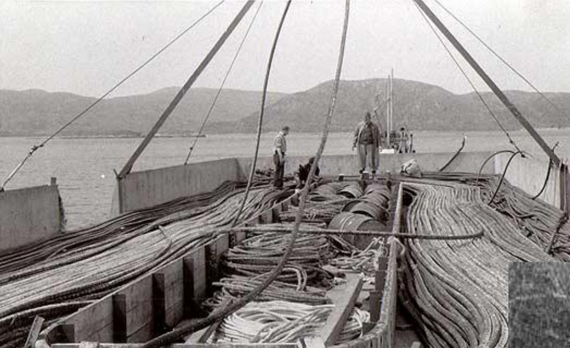
The TAT-1 Cable used for the transatlantic cable system on board the HMTS M
