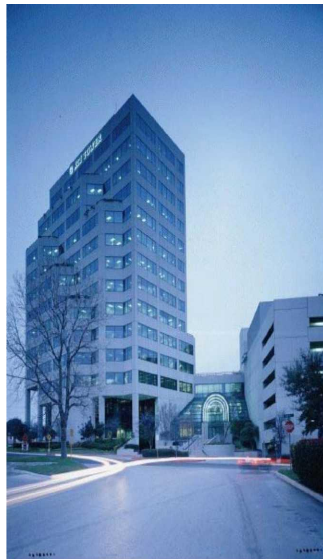
KCI Tower, San Antonio
