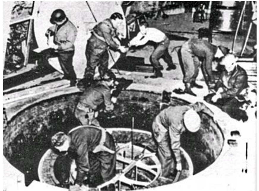
Nazi German experimental nuclear pile at Haigerloch
