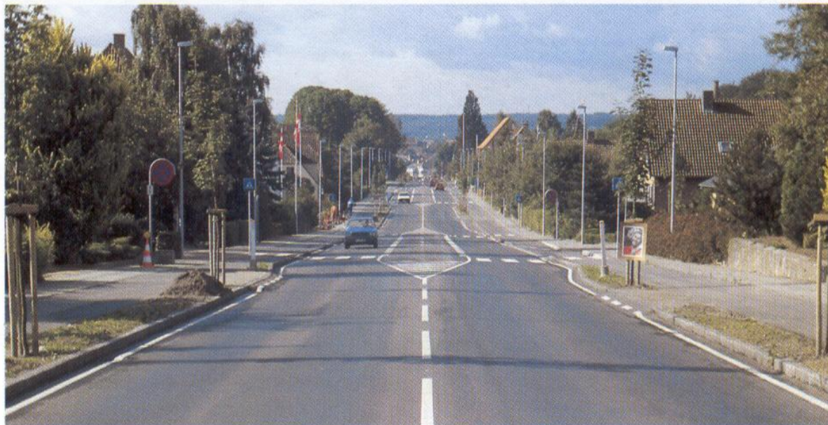
The traffic island shields off the left-turn lane and provides for safer crossing of the road.
