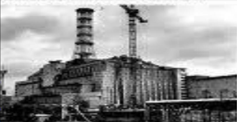
The reactor disaster in Chernobyl took place on April 26, 1986. The reactor was encased as a temporary solution to secure the site for only 20-30 years.
