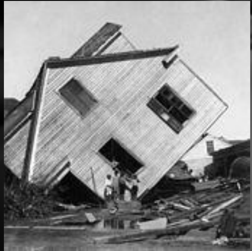
House in Galveston on Avenue N, October 15, 1900
