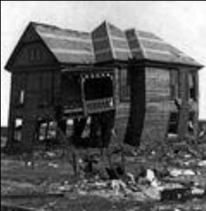
The only remaining house near the beach for miles, Galveston, Texas
