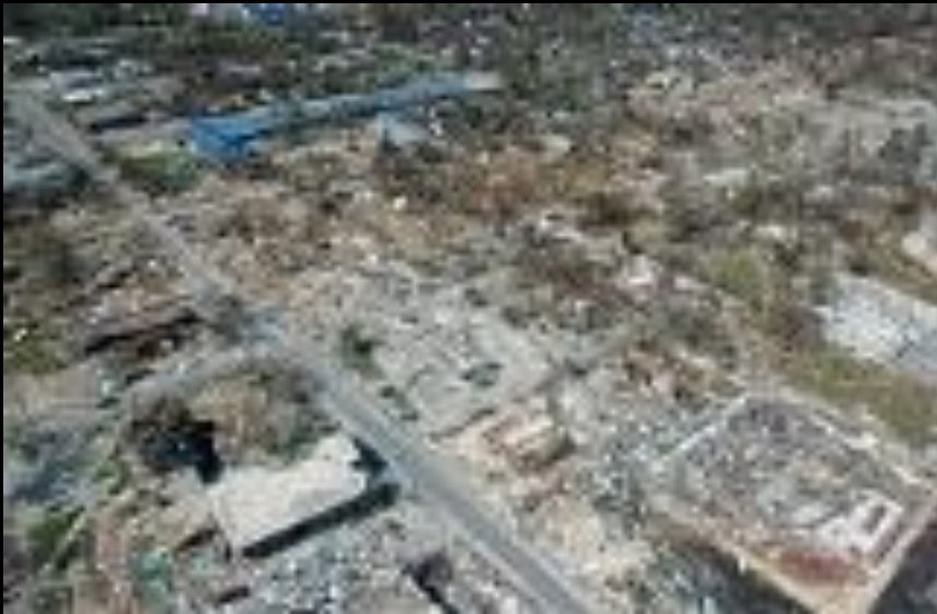
Damage to Long Beach, Mississippi following Hurricane Katrina
