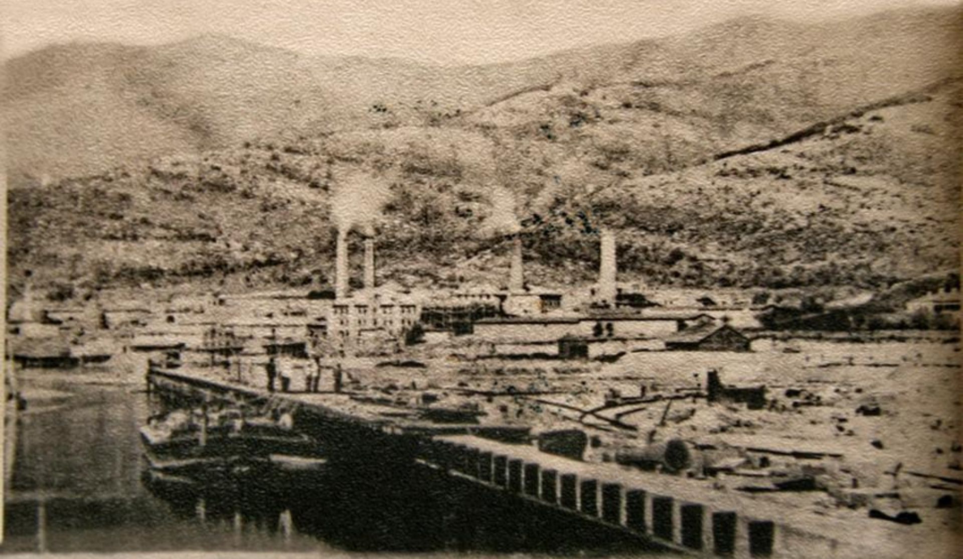
Цементный завод Черноморского О:ва при постройкѣ пристани The factory of cement of the Black-Sea-Company during the repair of the Loading-Stage
