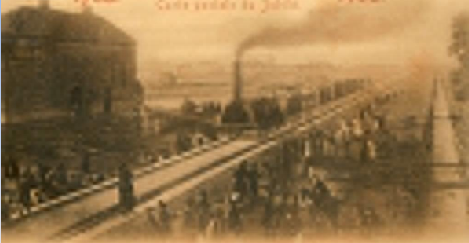
View of the factory from the street, 1900
