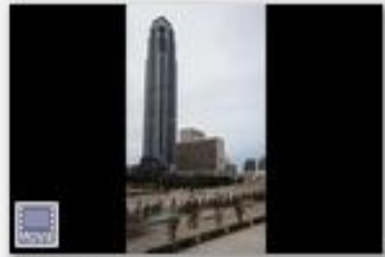
2008-02-06 Time Lapse Tower
