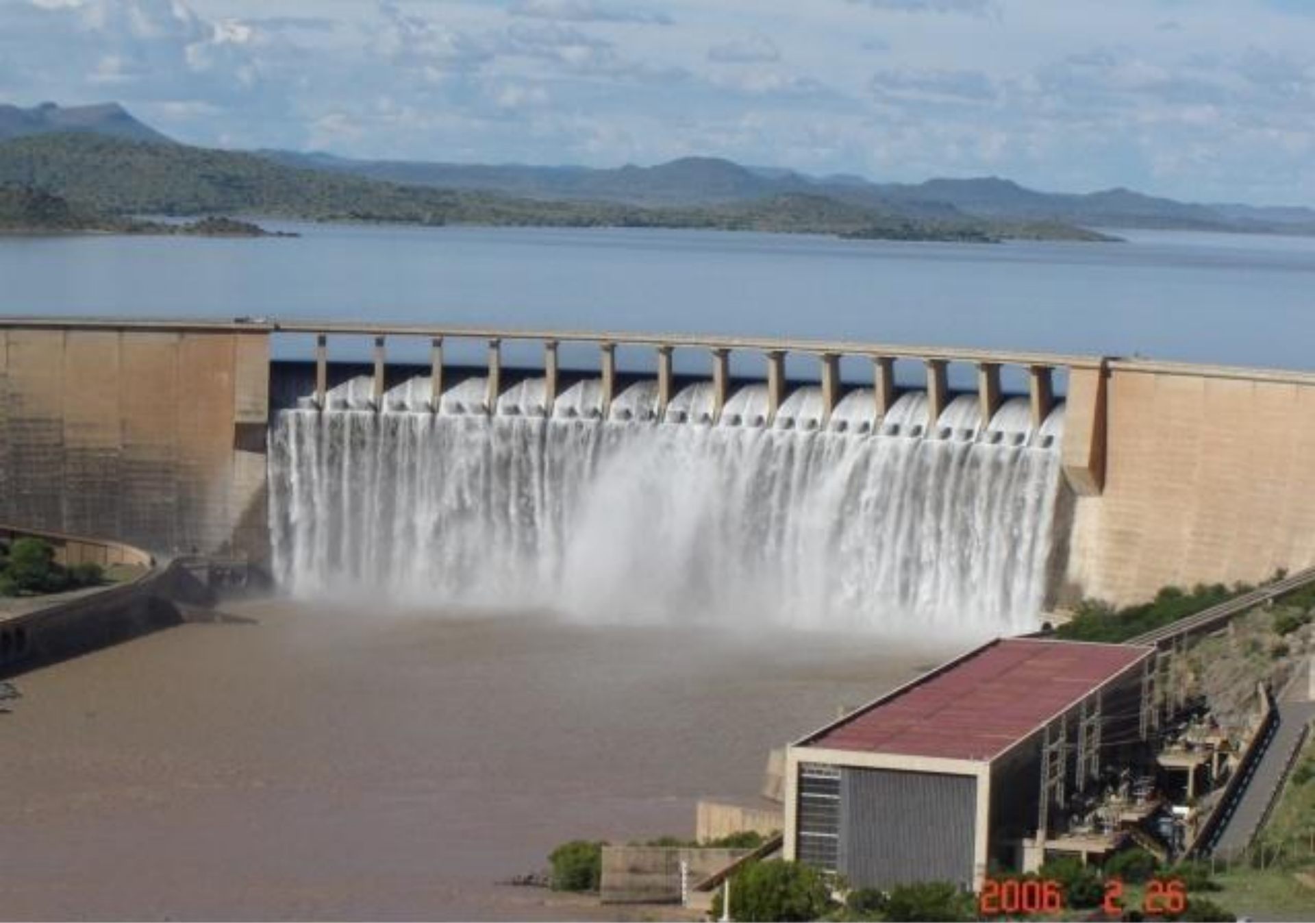
ESCOM Gariep Dam Aug 2006
